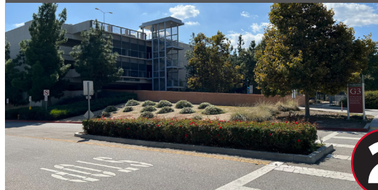
Parking Lot G3 Structure
